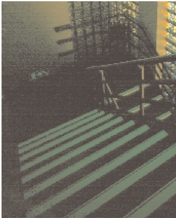
Shown at left, Johnsonite photoluminescent, visually impaired stair treads, photoluminescent hand rail covers and photoluminescent low-location signage with lights off.
